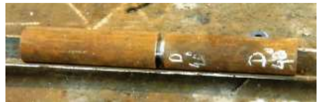
Fig.4 Edge preparation for welding
